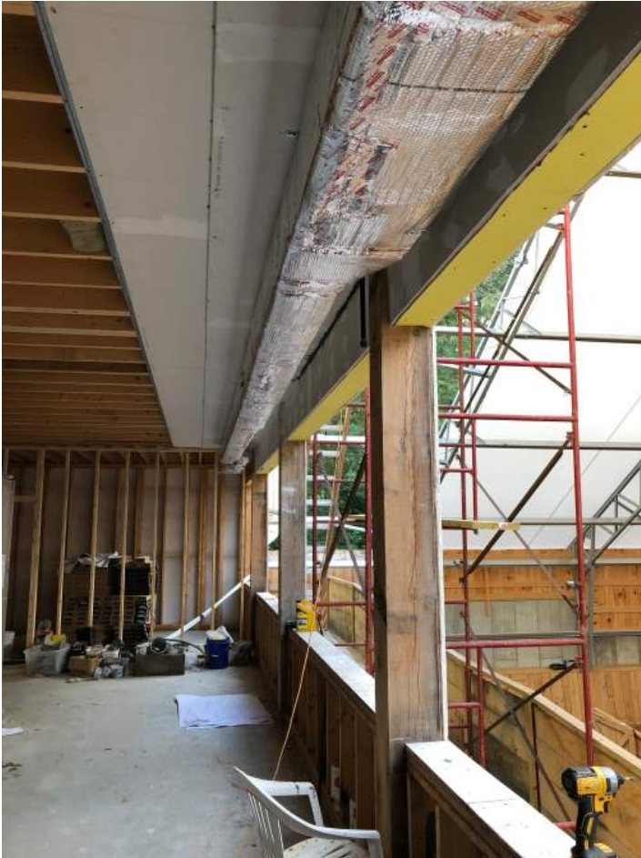
Mechanical ductwork is being installed at tack room.
