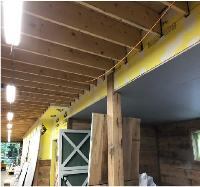
Interior drywall / 2-hour fire separation at underside of apartment egress deck - ongoing.
