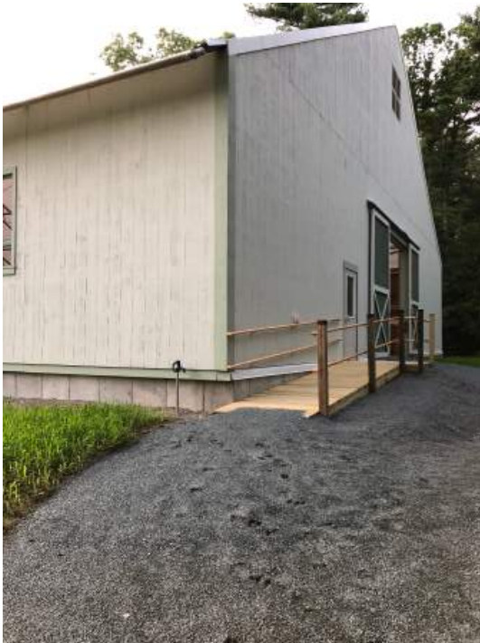
The accessible means of egress at the south end of the arena has been completed. The architect has conducted the final inspection and determined the project is substantially complete and ready for final inspection for the certificate of occupancy.
