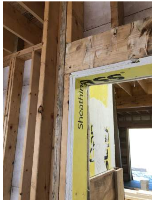
The 2 hour fire-rated floor / ceiling assembly between the apartment and tack room under construction.
