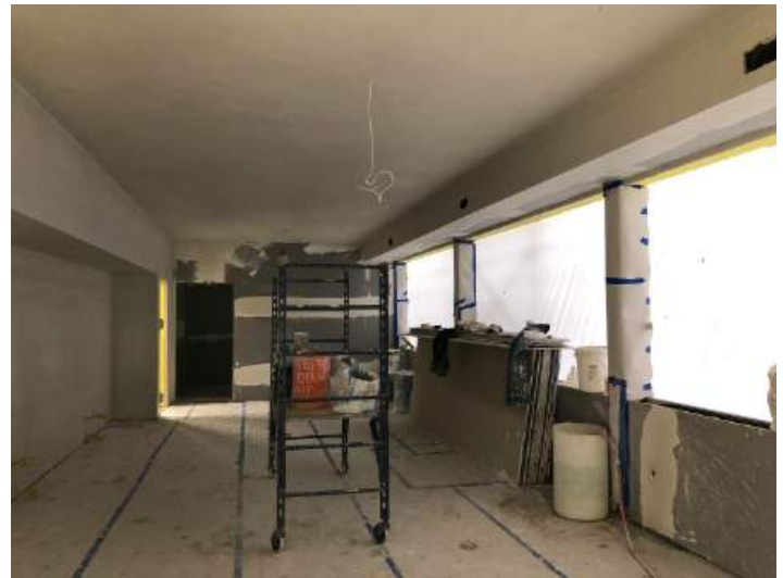
Interior drywall and veneer plastering at tack room, office and toilet / laundry - ongoing.
