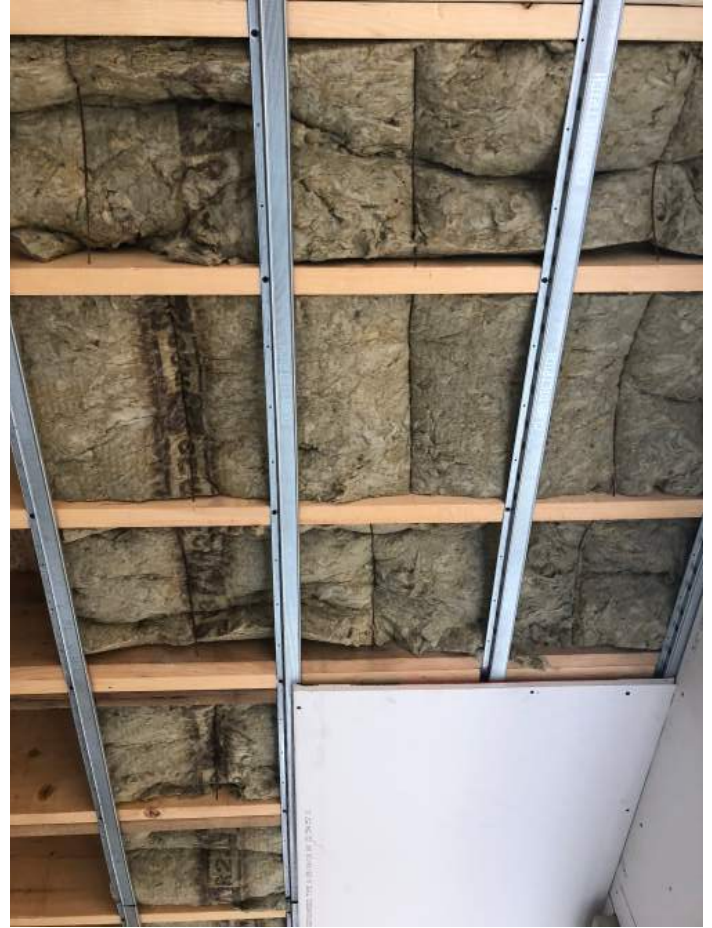
The 2 hour fire-rated floor / ceiling assembly between the apartment and tack room under construction.
