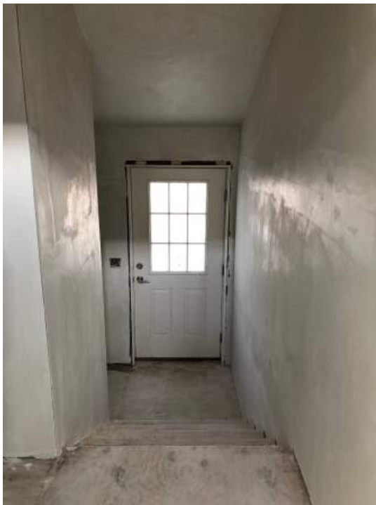
Veneer plastering is ongoing at apartment and rear egress stair.
