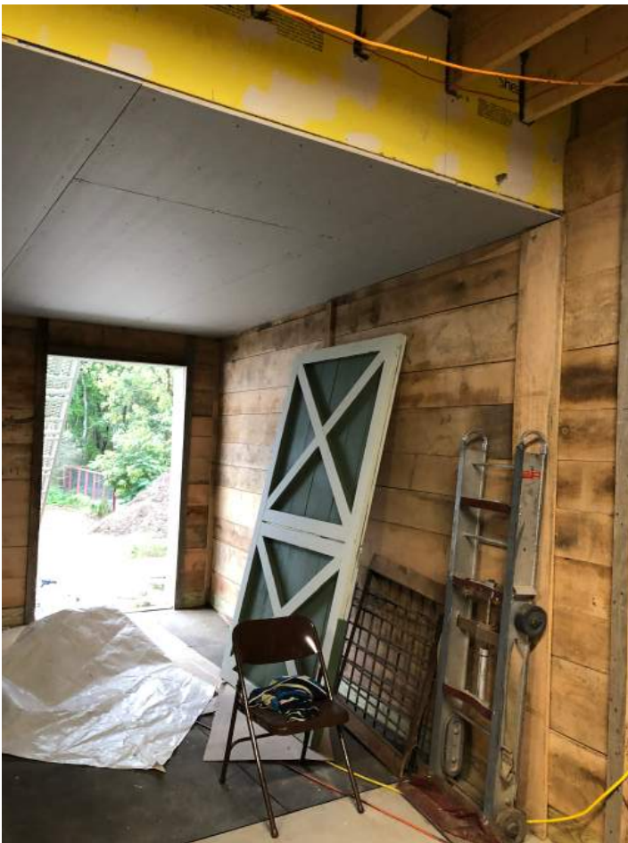
Interior drywall / 2-hour fire separation at underside of apartment egress deck - ongoing.
