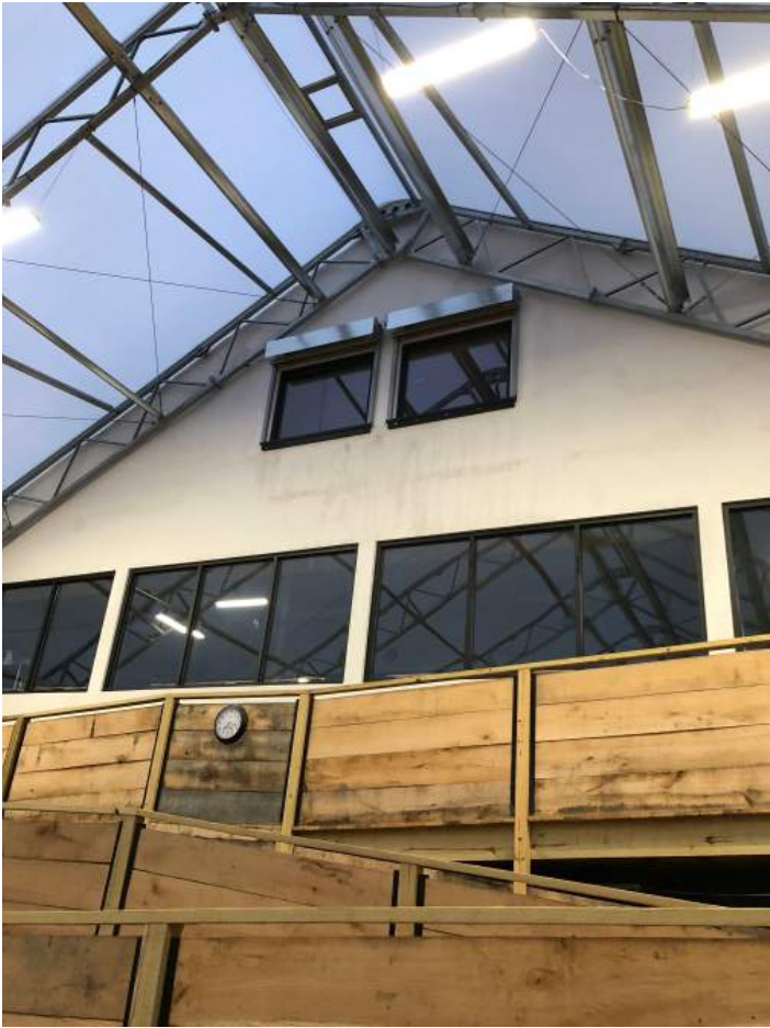
The non-rated windows and fire shutter from apartment to arena have been completed.
