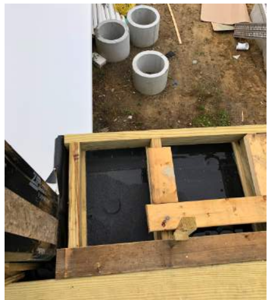
All components of 2-hour fire rated assembly at tack room are in place. This view is at door opening. Decking is being installed above the EPDM waterproofing membrane / sleepers at apartment egress deck (below).
