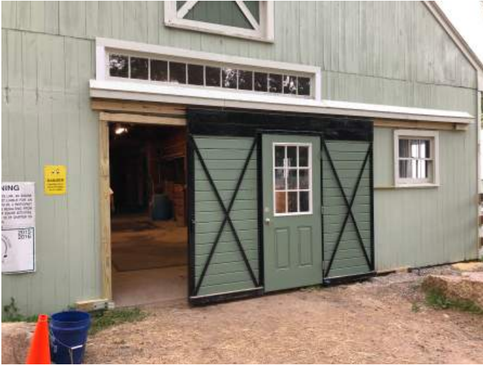
The new sliding door partially-opened with clear 34" dimension at left, and accessible man door positioned against limit of the existing barn aperture.
