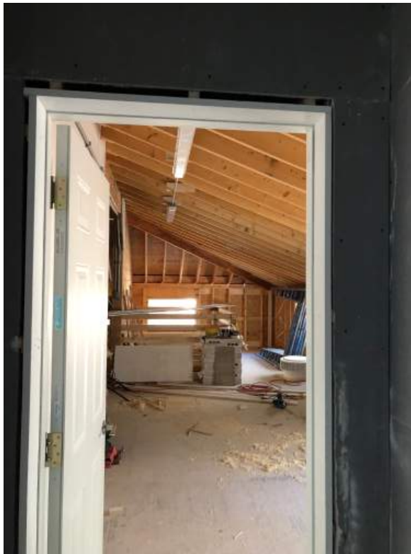
The B label doors are being installed at apartment and hay loft to exterior stairs.
