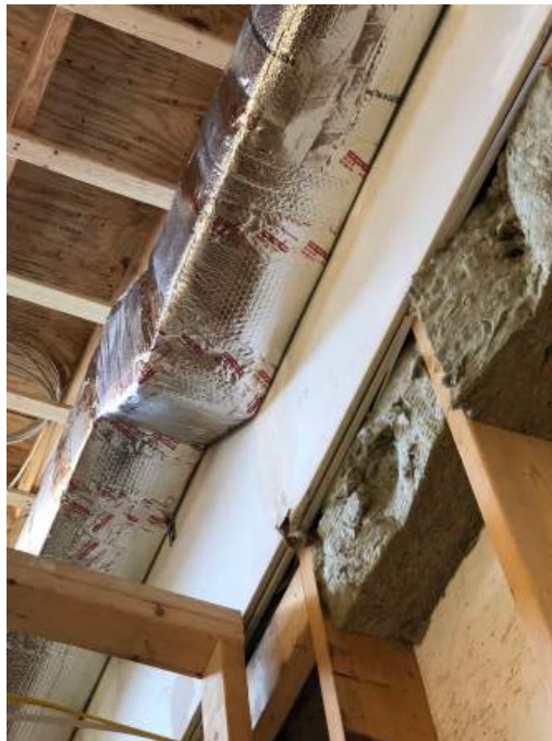
Apartment interior 2-hour rated partition is being completed on the apartment side. The perpendicular partitions are being held away from the two-layers of gypsum board.
