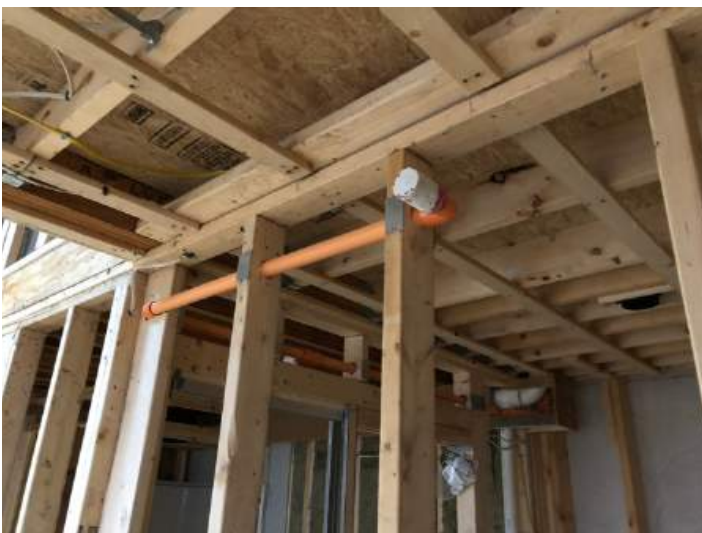
NFPA 13D system is being installed in apartment.
