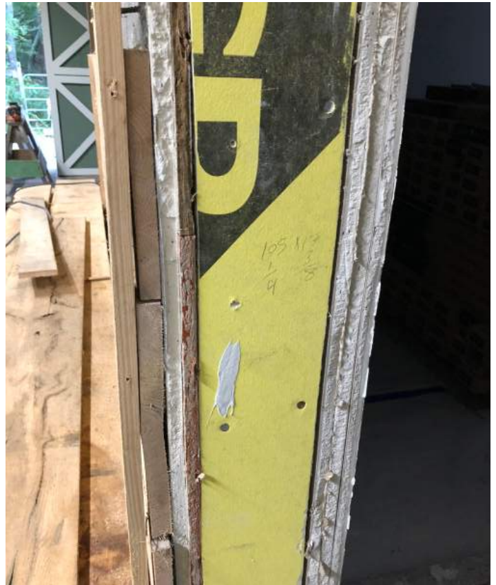
All components of 2-hour fire rated assembly at tack room are in place. This view is at door opening. Decking is being installed above the EPDM waterproofing membrane / sleepers at apartment egress deck (below).
