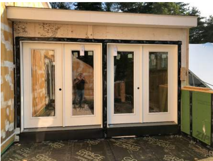
Apartment exterior doors and windows are being installed.
