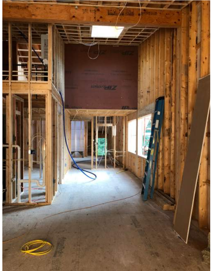
Apartment interior partitions have been framed.
