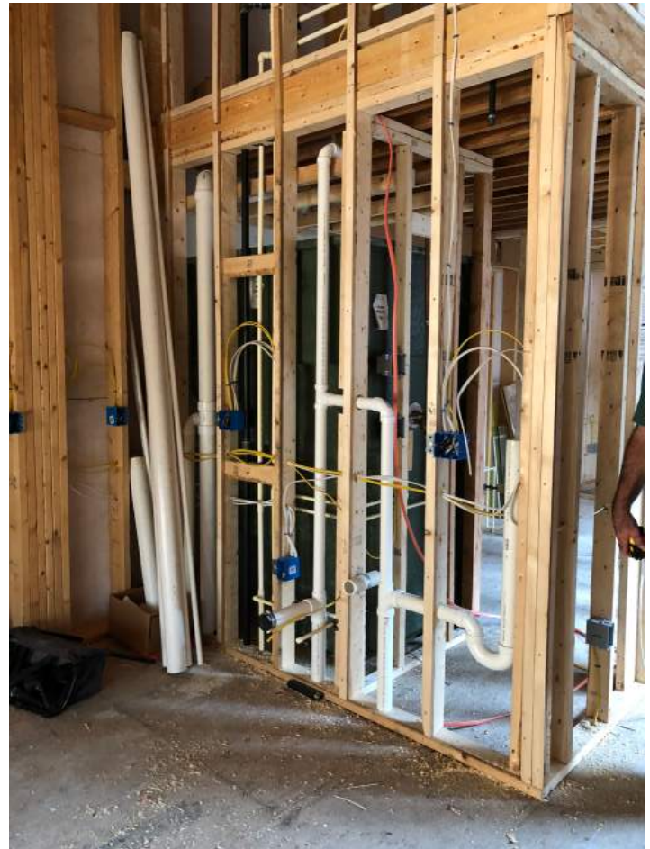
Plumbing and electrical rough-in ongoing at apartment.
