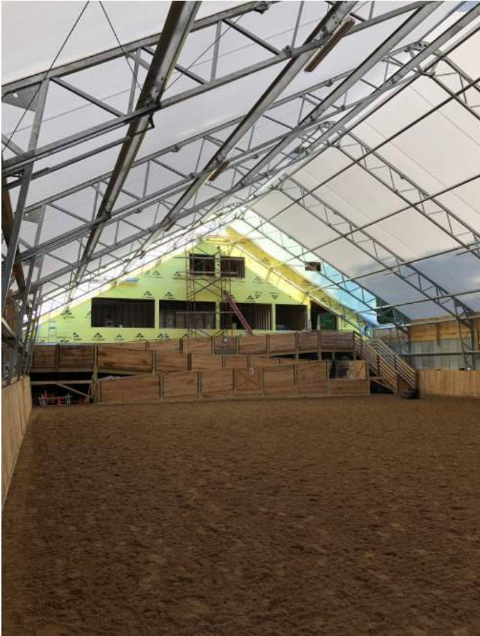
Storefront and windows at apartment have not been installed.
